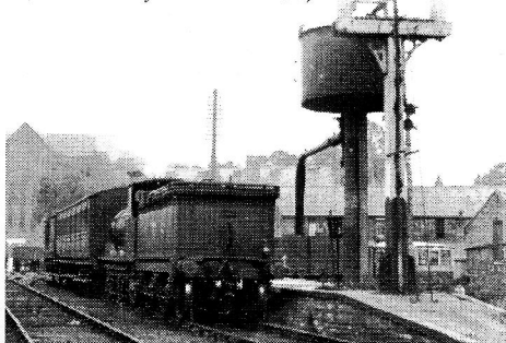
SMR Shrewsbury Abbey station showing water tank (Leslie Darbyshire Collection)
