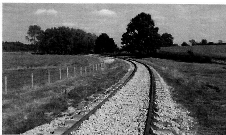
New track, ballast and fencing west of Bodiam. Photo: Mark Yonge
