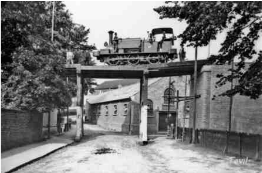
Is this the future Aldwyth crossing Church Green, Tovil, Kent ?
