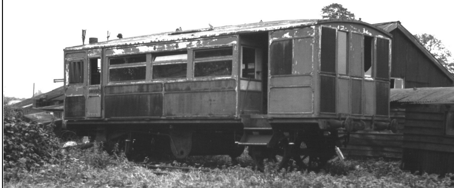
Number 6 in an advanced state of decay in Rolvenden yard, showing modified guard's end with just two windows.
