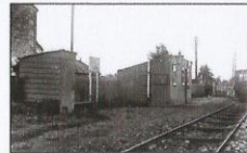
Worle Town Station looking towards Weston.
