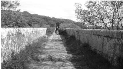
Treffry Viaduct is 648ft long with ten arches and is 98 feet high. It was the first large granite viaduct in Cornwall, began in 1839. The aqueduct channel runs below the trackbed.
