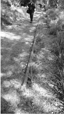
A section of wrought iron rail still insitu on Treffry's tramway complete with cast iron sleepers mounted on stone blocks.
