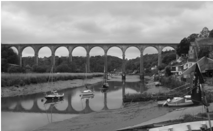
Calstock Quay and Viaduct showing the tidal nature of the Tamar.
