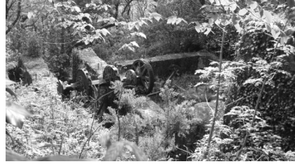
The Remains of the Thirty Foot Waterwheel that Allowed Loads to be Hauled up the Half Mile Long Incline from Pons Mill.
