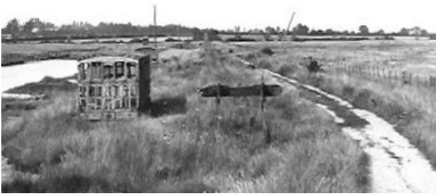
Site of Tollesbury Pier Extension circa 1930. Ralph Gillam Collection
